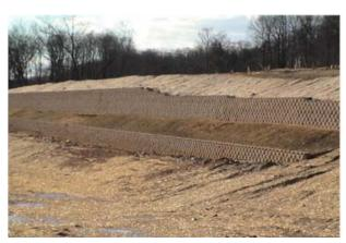
Figure 5.1-6. Woodland removal for steep slope development with retaining walls
