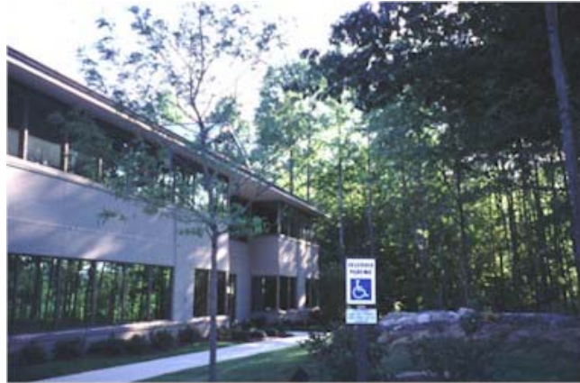
Figure 5.6-3 Woodlands Protected through Minimum Disturbance Practices
