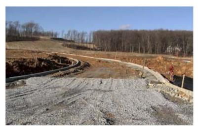
Figure 5.7-2 Example of site development with extreme soil compaction on steep slope
